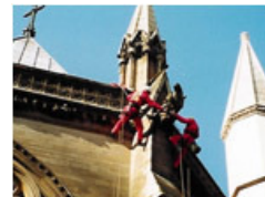
Westminster Abbey Safety survey and protective netting installation on stone gargoyles.
